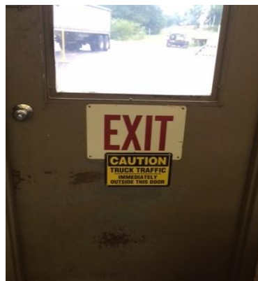
*barricades can protect stationary employees as well as guide them to a desired route, signage warns of exits leading into traffic areas.
